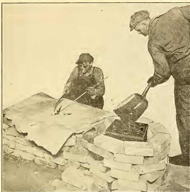
FIG. 135.—Welding and Preheating.
